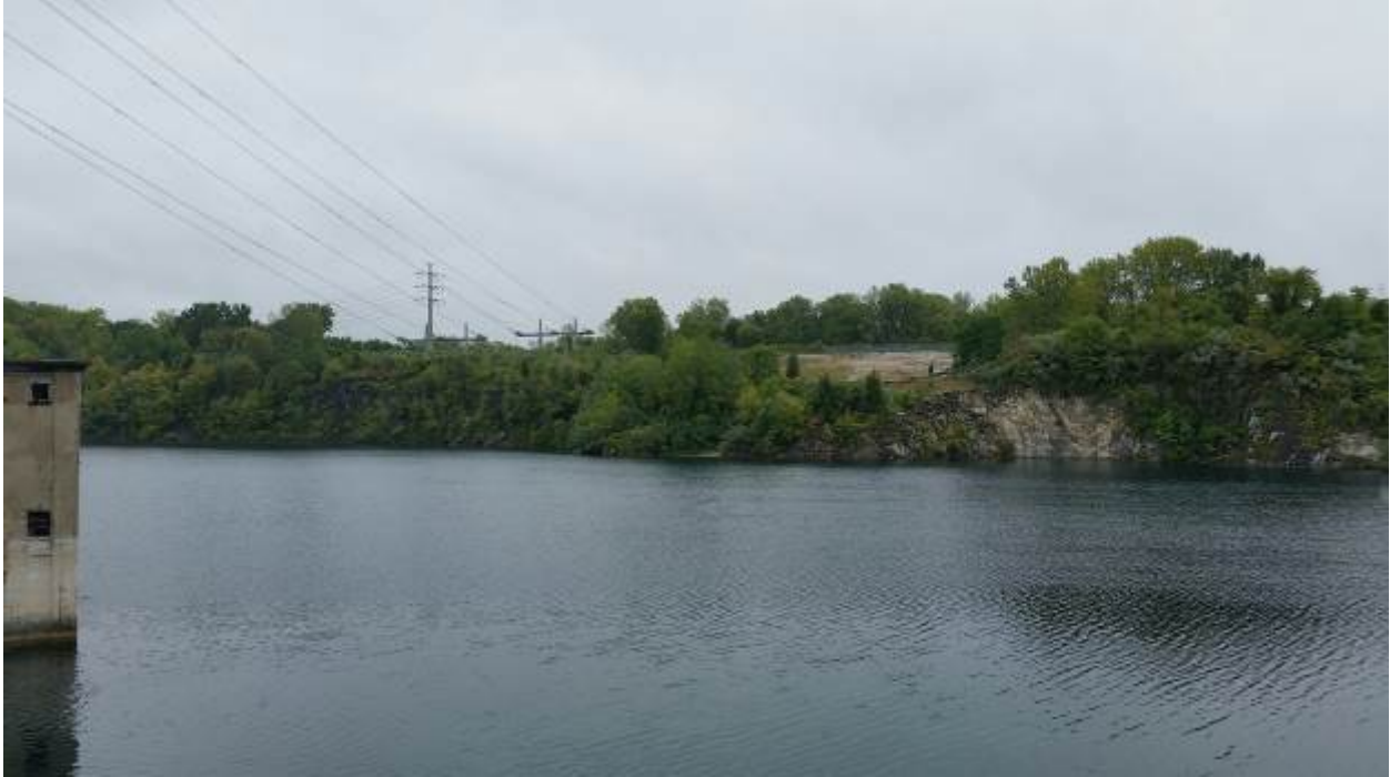
SEPTEMBER 28, 2016 – CON EDISON AERIAL WIRES ACROSS QUARRY
