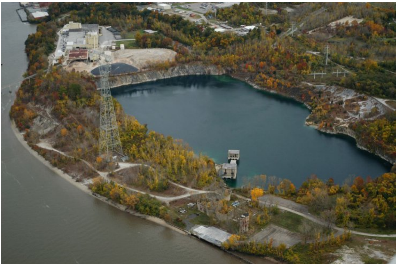
Aerial View of former Con Edison Property and Verplanck Quarry
