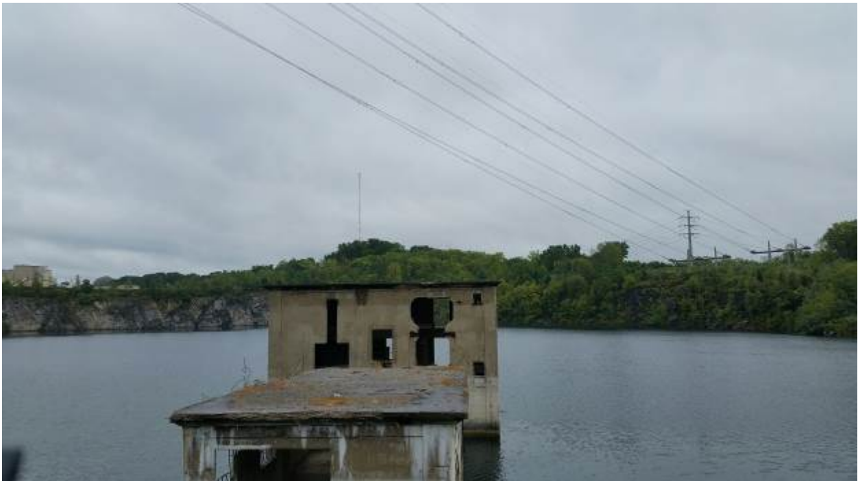
SEPTEMBER 28, 2016 – QUARRY BUILDINGS LOOKING NORTH EAST
