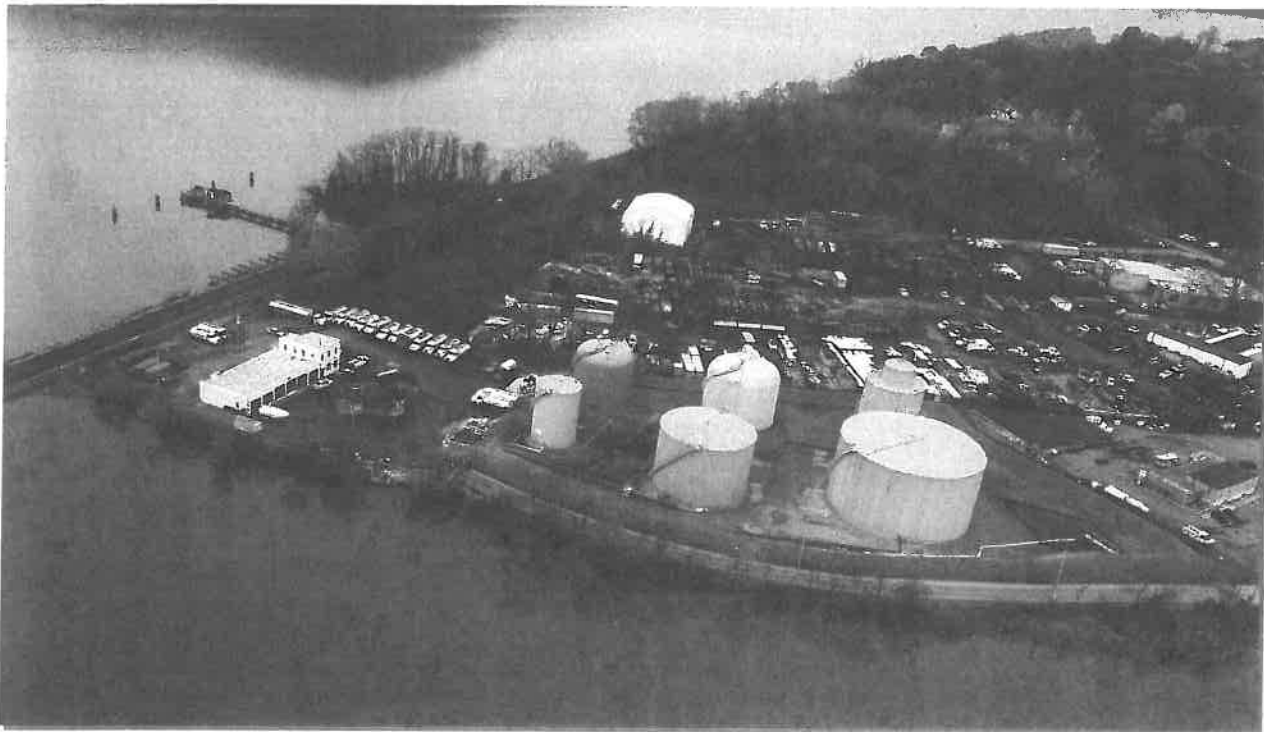
Figure: Meenan Oil – along the Hudson River, view looking north (4/24/2017)
