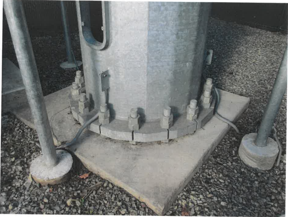
Photo 3: Pole Base and ground leads
