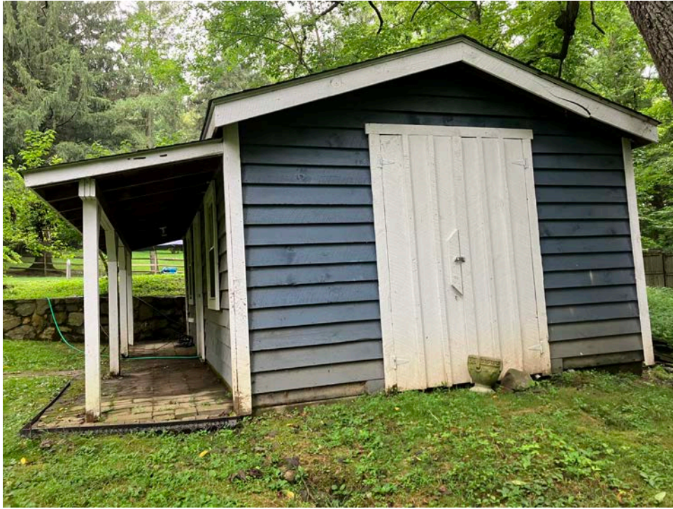
Accessory Structure View of Exterior at Side
