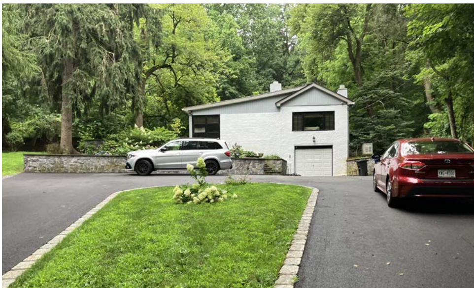
Principal Building View of Exterior
