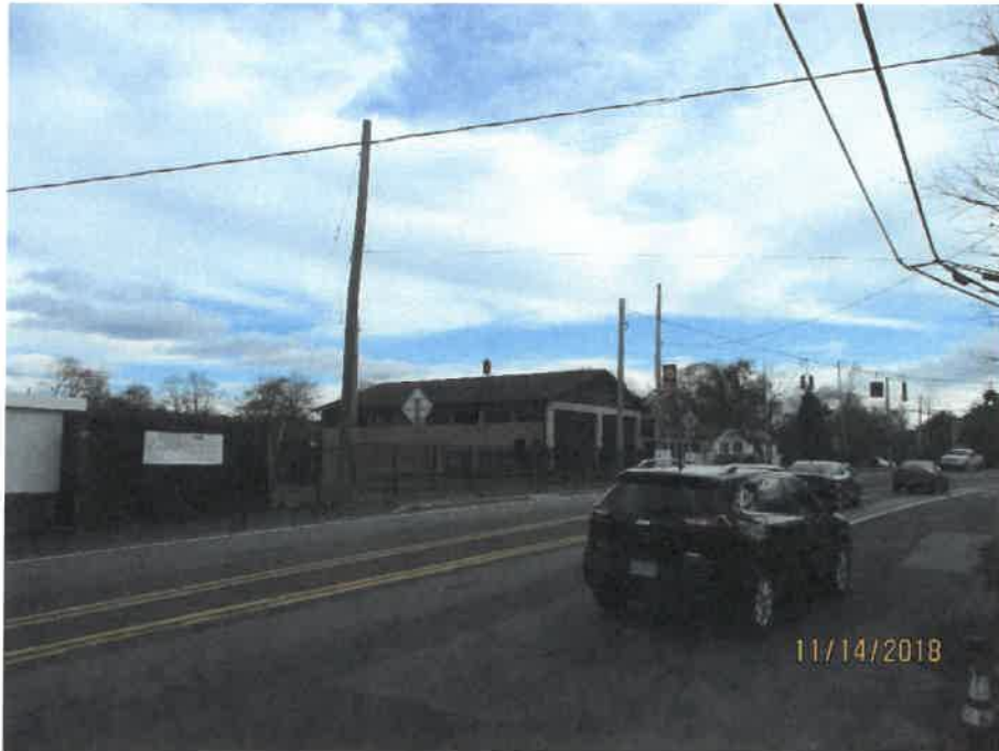
Photo 4: Existing View Looking Southeast on Albany Post Road
