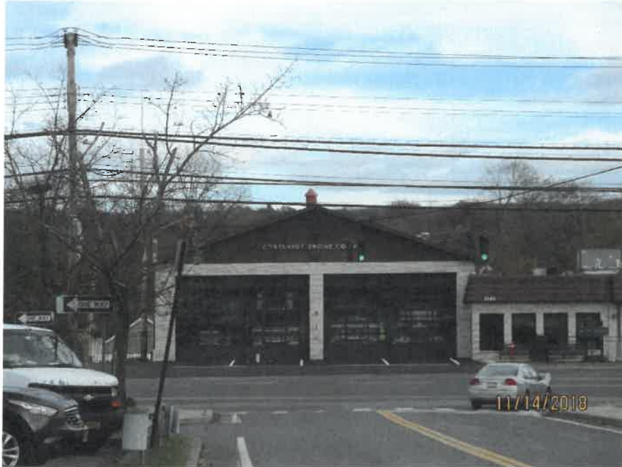
Photo 1: Existing View Looking East on Kings Ferry Road
