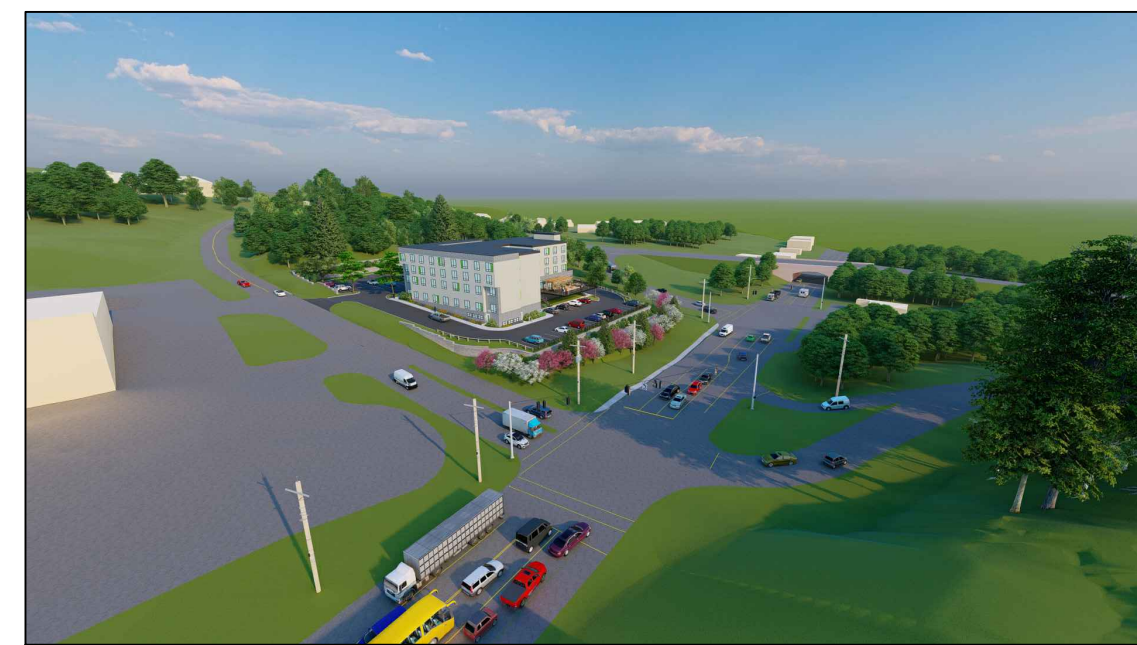
21 BIRDSEYE - DOWN E. MAIN STREET L1.4 FACING NORTHEAST
