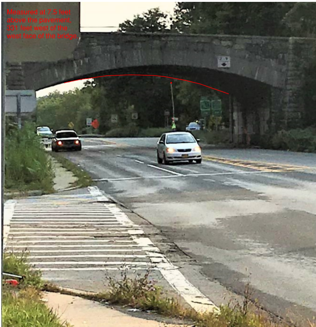
Red Signal Head Centered 19' over the roadway, when viewed from 7.5 feet over the Roadway
