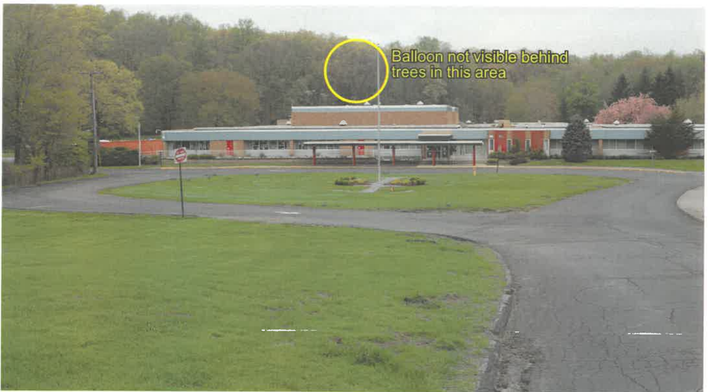
VP24 - Watch Hill Road near Furnace Woods Elementary School
