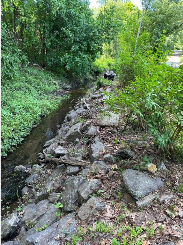
Photo 1 Looking south along reinforced stream
