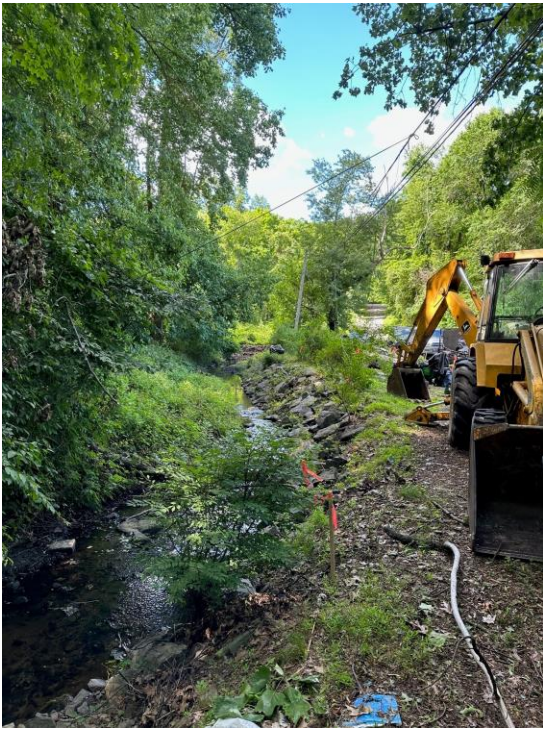
Photo 5 Looking south downstream along east side of site
