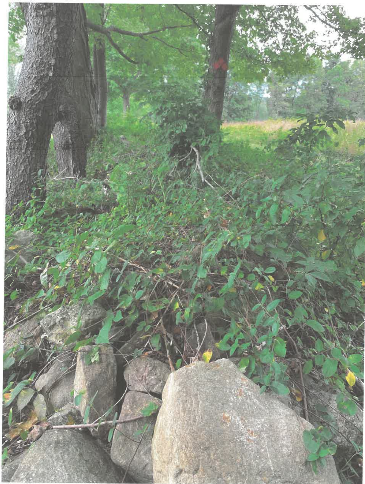
Figure 4. Hedgerow 1, overgrown with invasive vines, nearest Teatown Rd.
