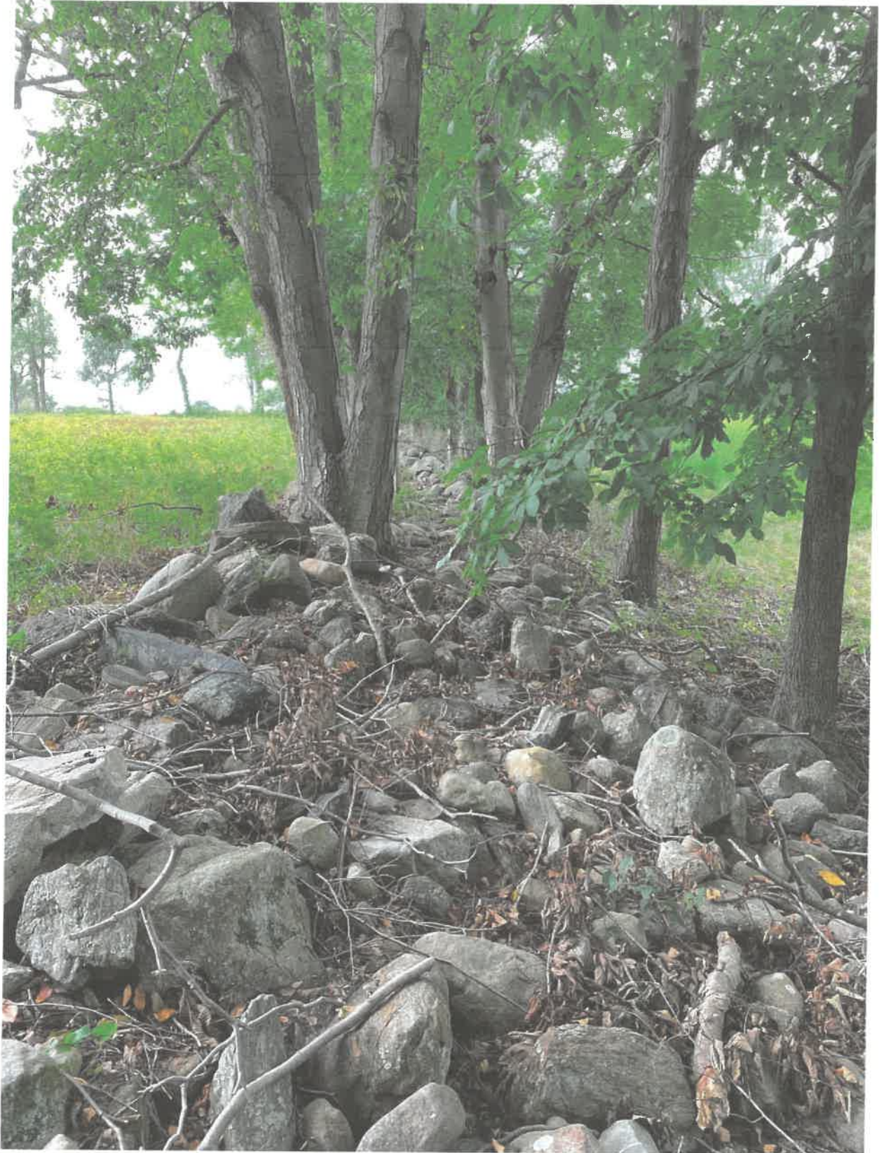
Figure 1. Hedgerow 2, far edge boundary for removal. Stone wall in poor condition.
