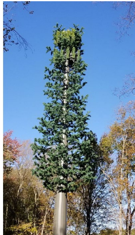
Example of a 120-ft tall Homeland Tower stealth tree monopole design with two arrays.
