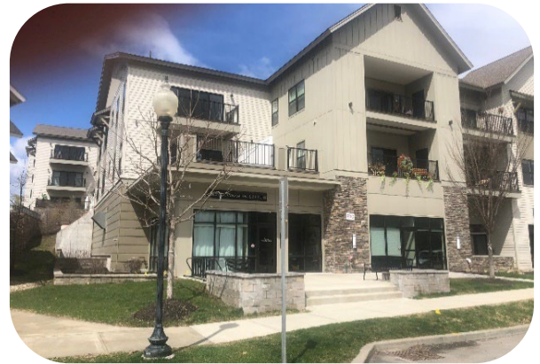
Three story mixed use building.
