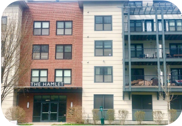
Four story plus penthouse mixed use building.
