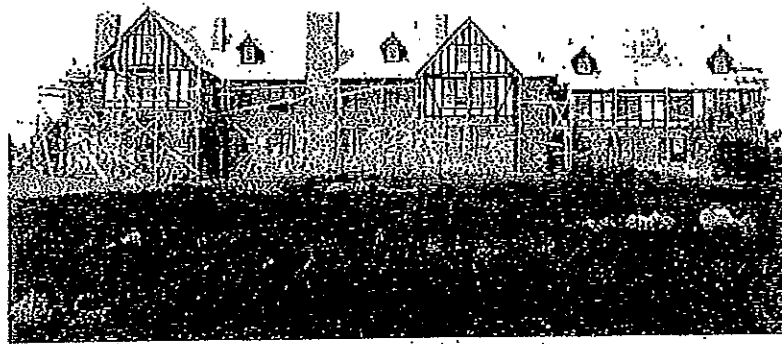
CONSTRUCTION OF THE MAIN BUILDING 1920-1922
