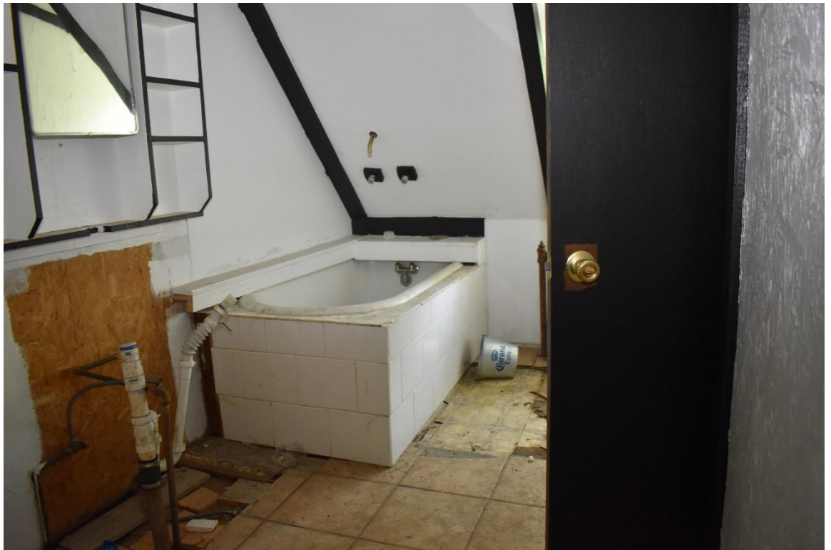
13. Bathroom on second floor. View to the southwest.
