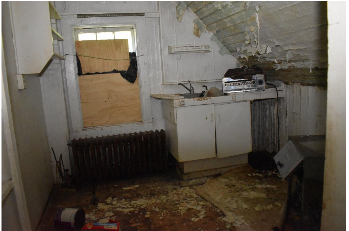
15. View to the west of the northern dormer and addition on second floor. Shiplap to the right in photos is collapsing inward.
