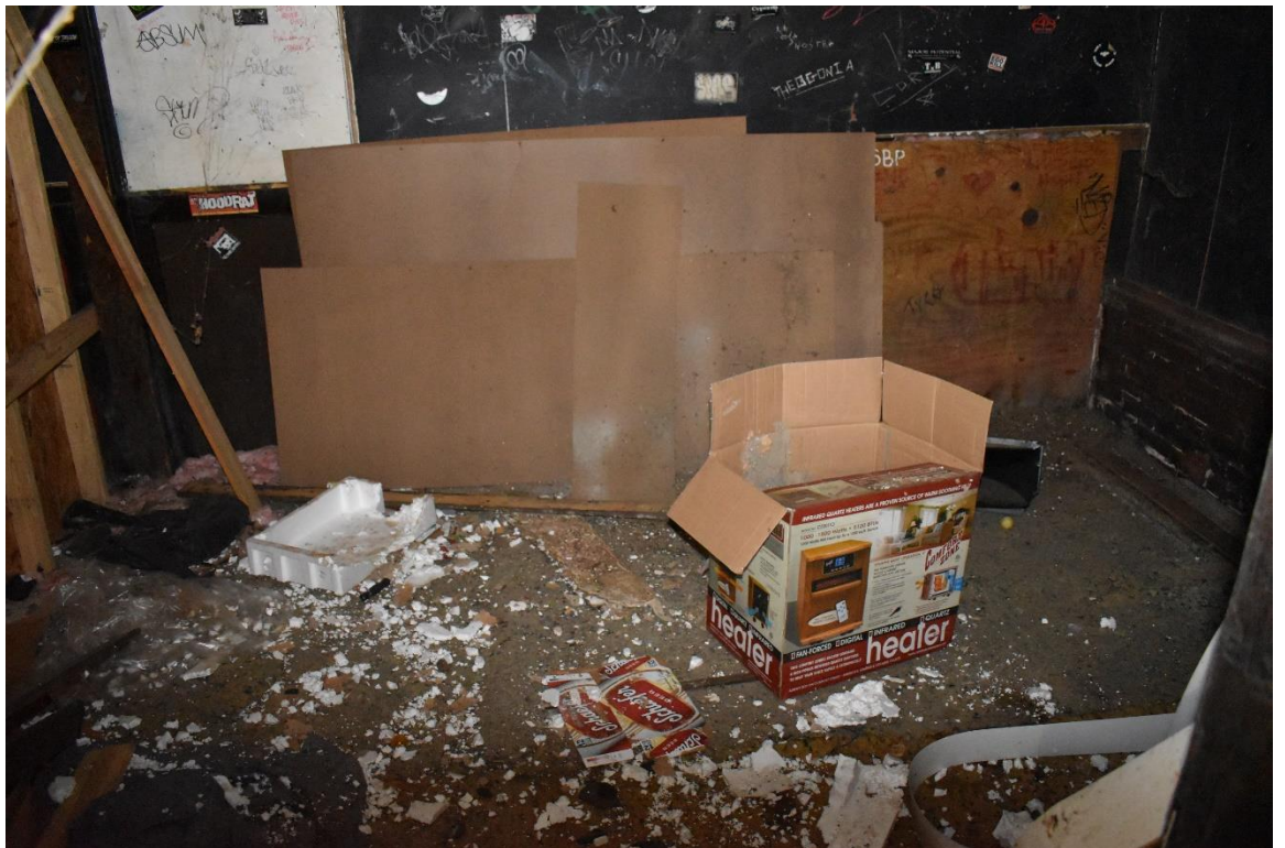
8. View to the west of the northern addition.
