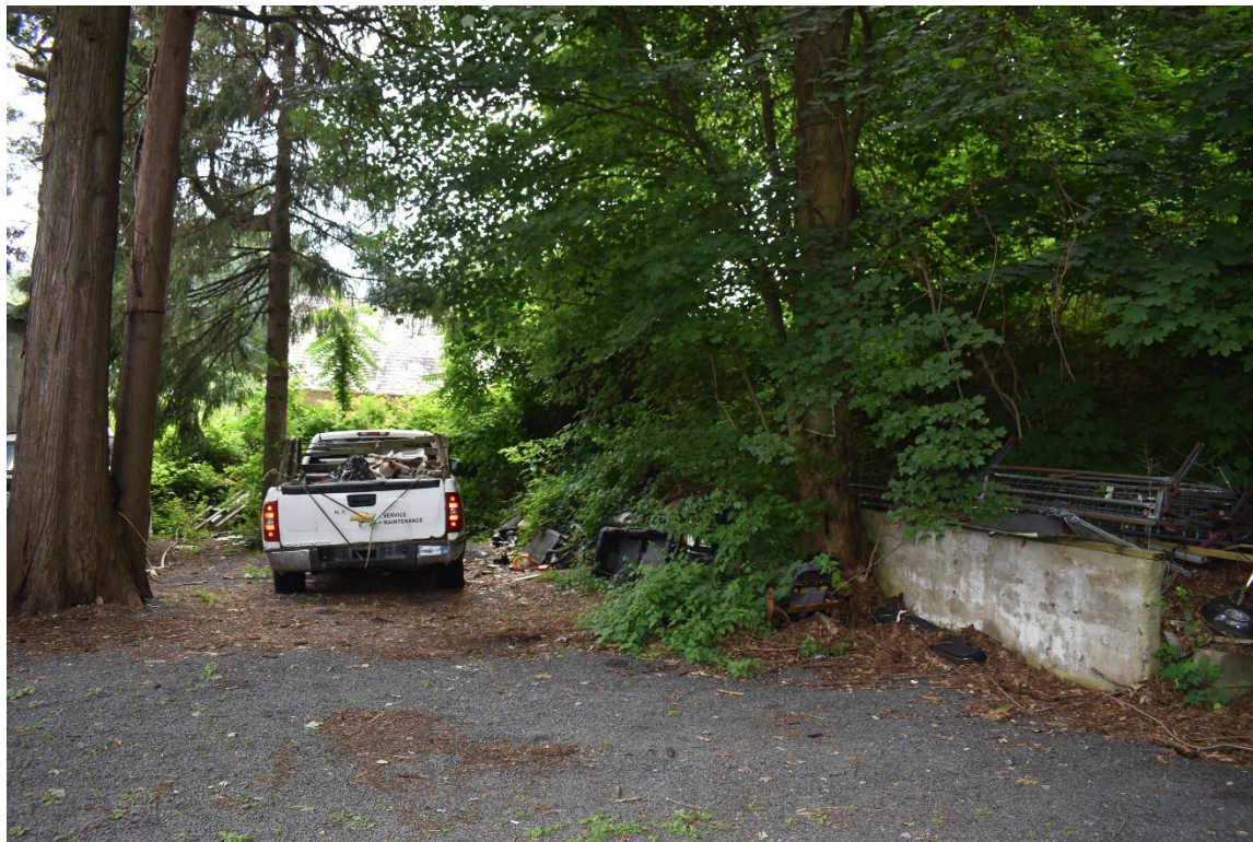
Photo 14: Retaining walls border the lot to the north (behind) the auto repair shop. View to the west.
