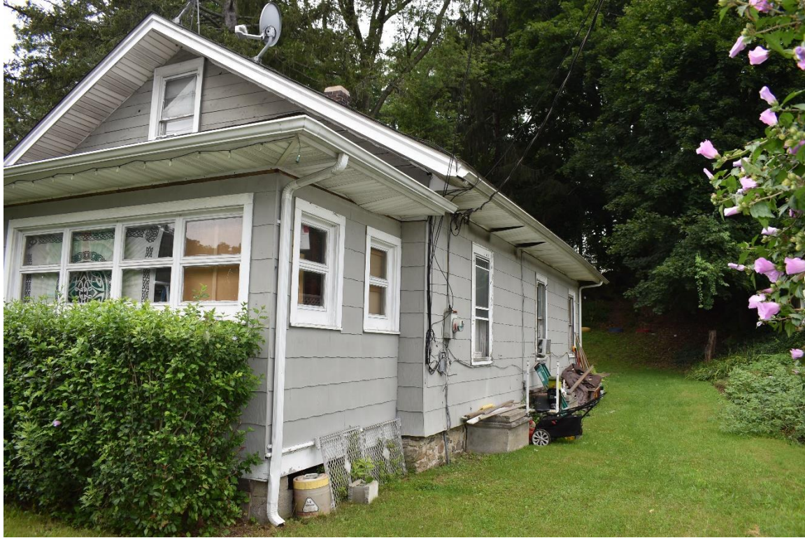
Photo 3: A wood frame residential structure is located in the northern corner of the Project Parcel. View to the northwest.
