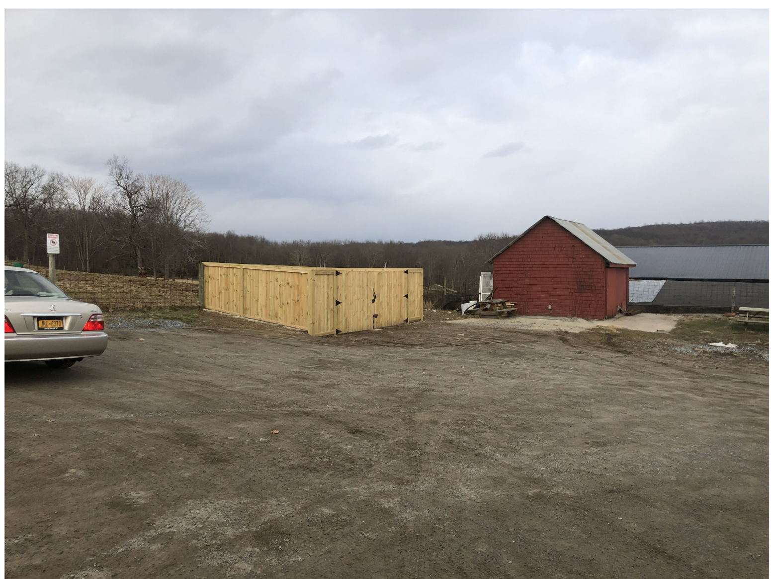
EXISTING PARKING LOT AND TRASH STORAGE
