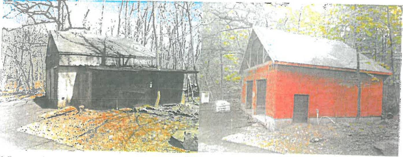
View of old barn/partially constructed garage. Note substantially similar footprint.
