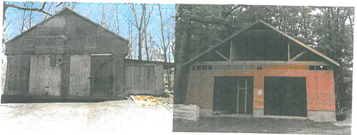
View of old barn/partially constructed garage. Note, substantially similar height, with slight shift in roof design to cover complete structure.
