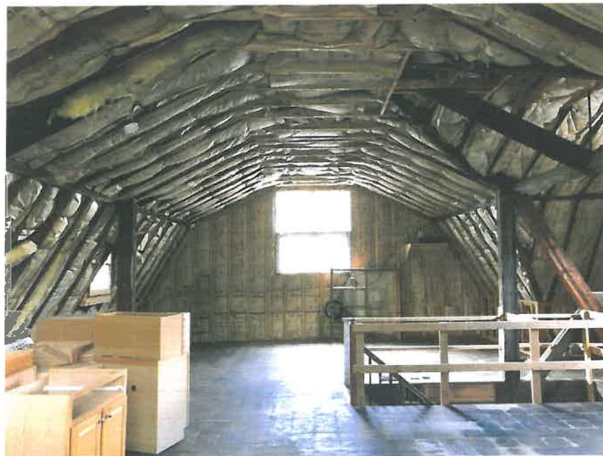
Current Interior of 2 nd Floor Loft
