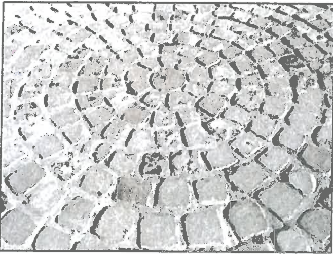
Cobblestones and other rough surfaces make wheelchair travel difficult and uncomfortable.
